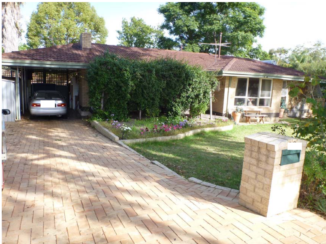
Front elevation of the inspected property
