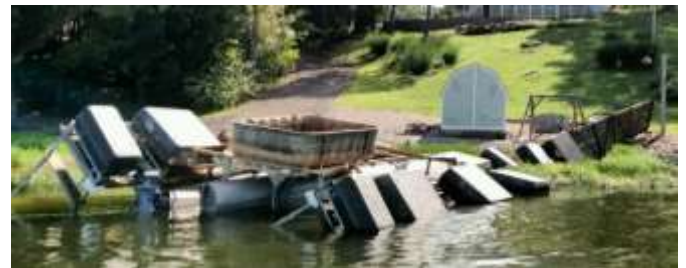
The above floating dock was flipped upside down, with the pontoon boat visible under the large floatation.
