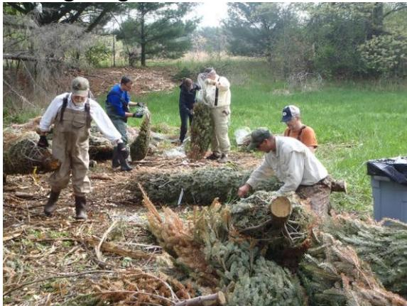
Unsold, dead and discarded Christmas trees are a valuable resource in this project. With the guidance of the DNR team, stakes are driven defining an area of the river to be filled in. Trees, which were floated from the stockpile to the work area in a johnboat, are then stacked on the stakes and woven together forming a wall and platform.
