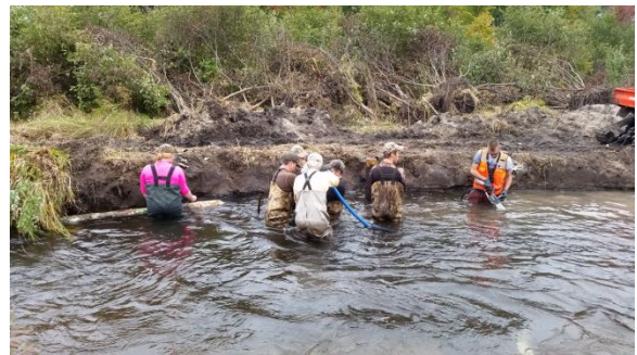
DNR Crew and Volunteers Jetting in Pilings for Stream Bank Structures
