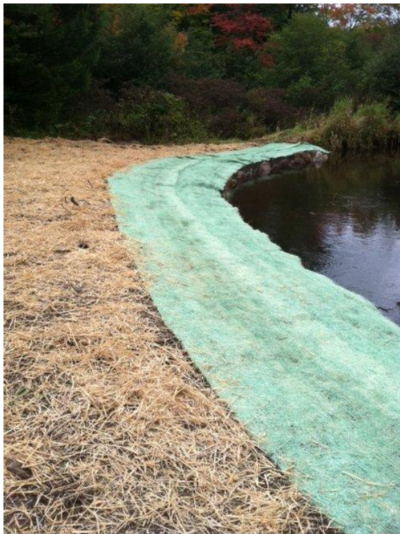
Finished bank cover
