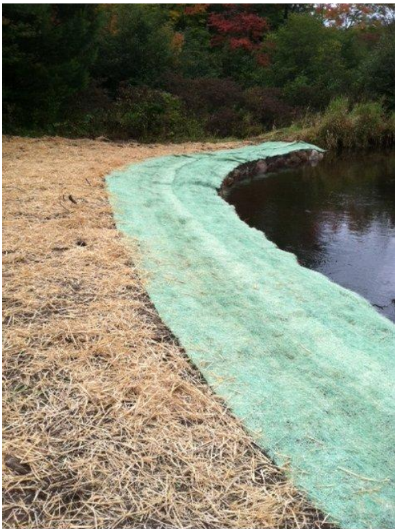
Finished bank cover
