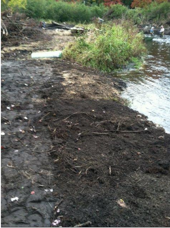
Preparing bank for seeding
